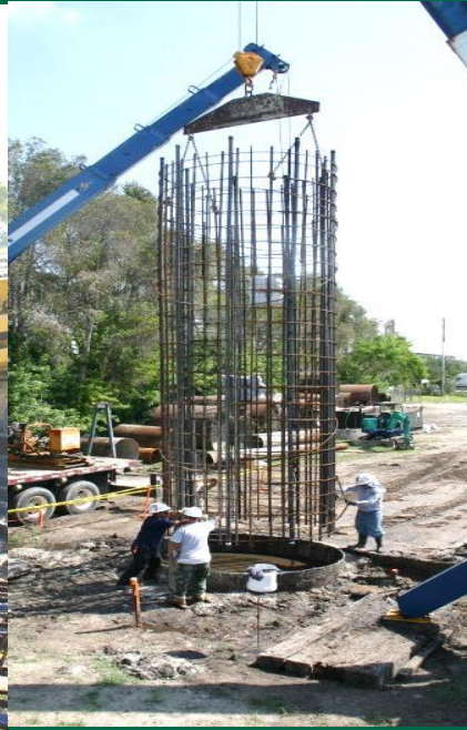
Placing rebar
