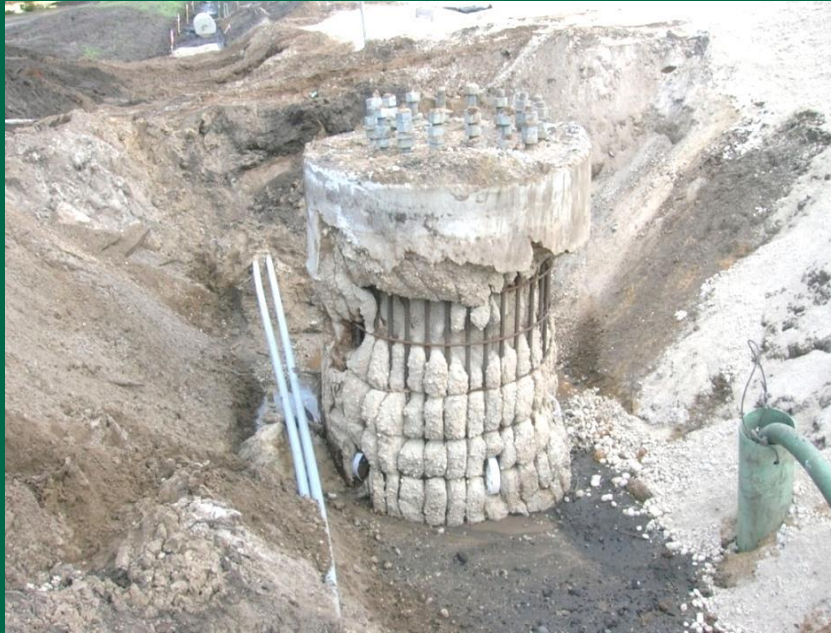
Shaft exhumed -poor concrete flow performance
