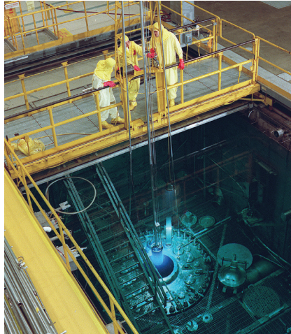
FIGURE 1. Technicians replace a fuel element of the HFIR at ORNL. The HFIR has operated since 1966 (over 452 fuel cycles) and is currently the only operating nuclear reactor at ORNL. Image courtesy of the Oak Ridge National Laboratory, U.S. Dept. of Energy.
