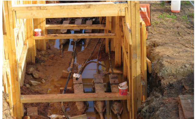
Figure 5. Photos of field joints being used to connect separate sections of cables together.
